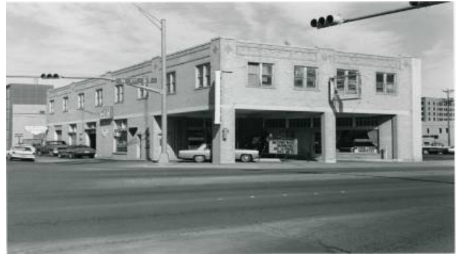
Boyd Building in 1992 (NRHP Registration Form)
