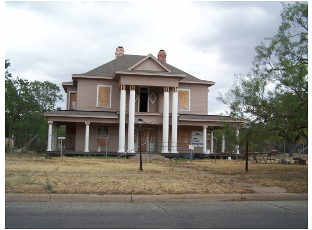
Stabilized and ready for rehabilitation 2012
