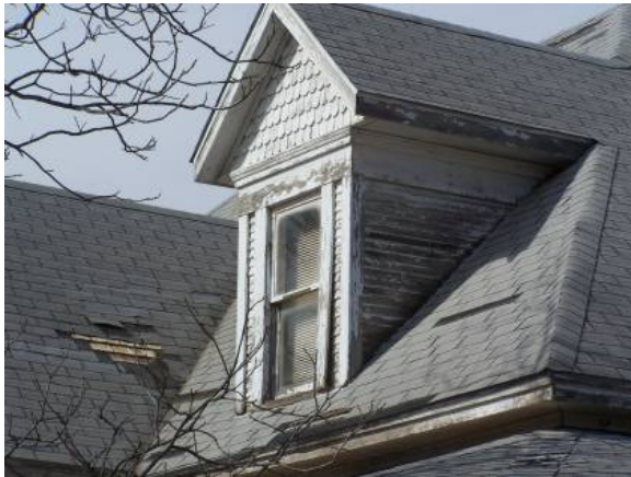
Close-up of dormer with shake roof visible in rear.
