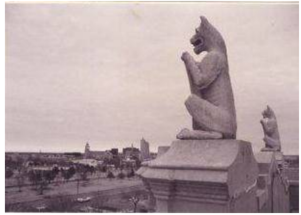
Lioness Gargoyles on roof overlooking 1st Street and the railroad tracks
